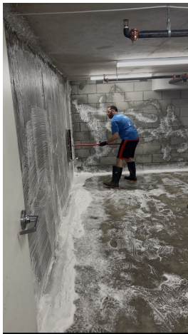
Manual brushing of walls and concrete-block joints.
