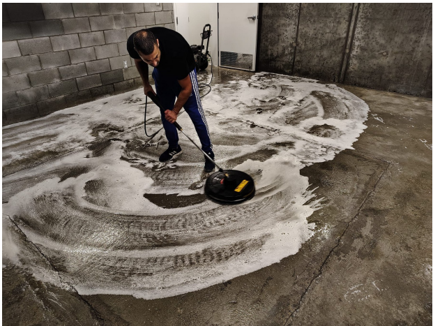
Mechanized pass over larger areas to loosen embedded deposits.
