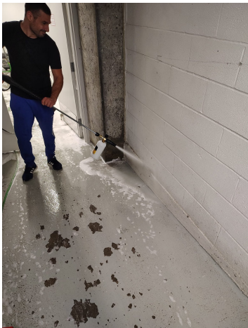
Cleaning solution applied to traffic areas and contaminated surfaces.
