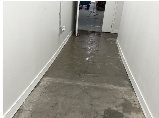
Technical corridor rinsed, disinfected, treated for odours and evacuated after the work.
