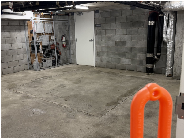
General view after intervention: rinsed floor, cleared surfaces and odours eliminated.
