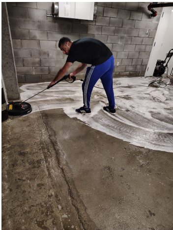
Uniform mechanical action over exposed concrete areas.
